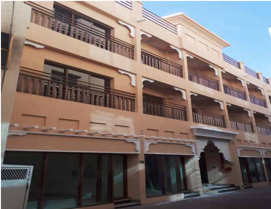
Project : G+M+1+R Building Consultant : Al Hutaib engineering Consultants
