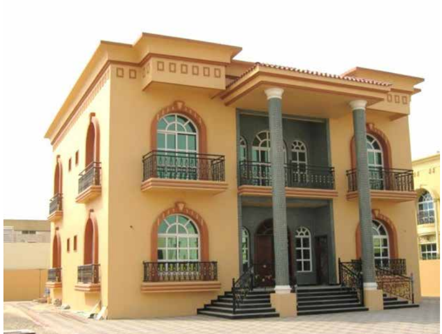
Project : G+1 Floor Villa Consultant : Arabian Modern Engineering Consultants
