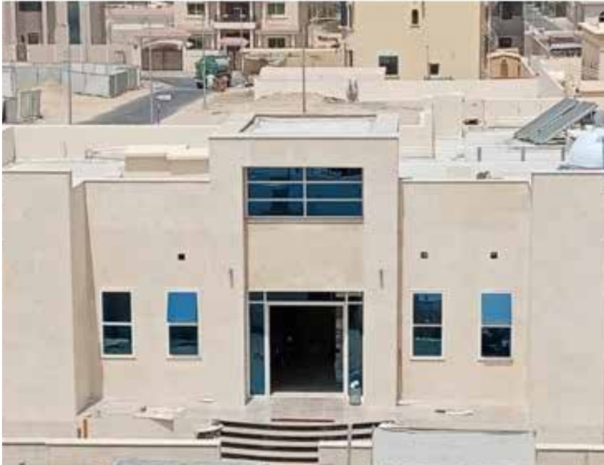
Project : G floor Villa with Service block Consultant : Red Crystal engineering consultancy
