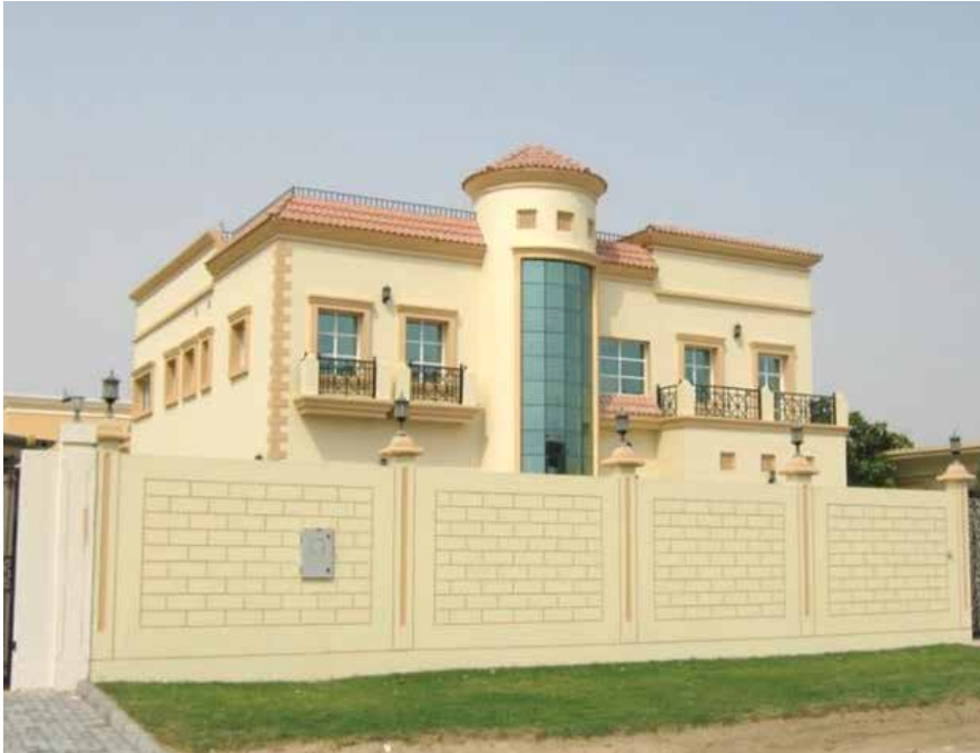
Project : G+1 Floor Villa with Outhouse Consultant : Chawla Architectural And Consulting Engineers
