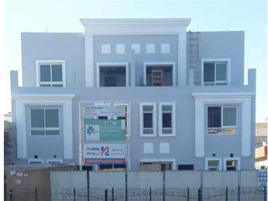
Project : G+F+R Floors Twin villa Consultant : Al Badiya engineering consultants
