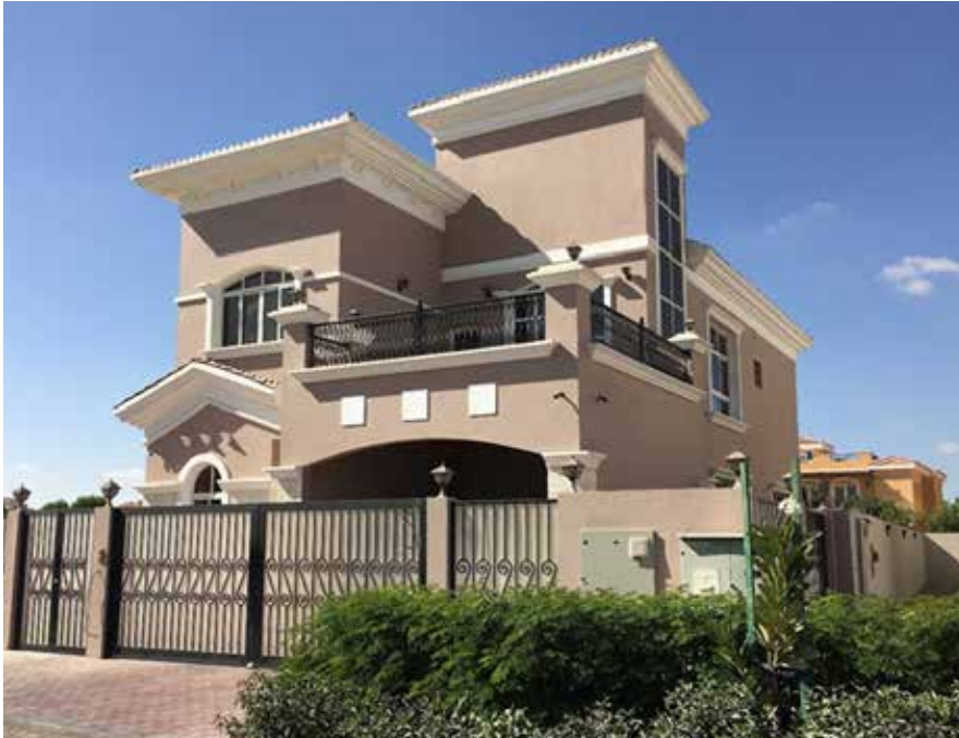
Project : G+1 villa Consultant : Emsquare engineering consultants
